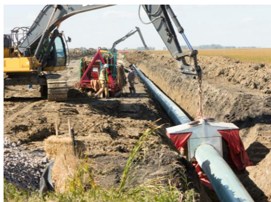
Line 3 Replacement Construction – North Dakota
