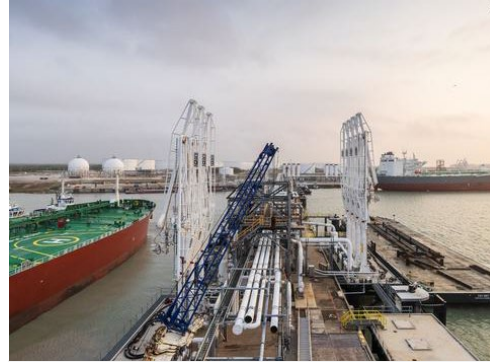
Ingleside Blue Hydrogen & Ammonia export facility showcases value chain integration
