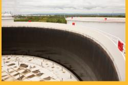
Crude oil storage terminals have built-in safety including computerized and manual shut-off valves for the piping and manifold systems, containment dikes around the tanks and floating roofs that minimize evaporation and capture emissions from the stored crude oil.
