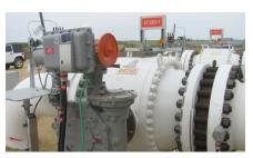
Motor operated ball valves allow our control staff to remotely close sections of our pipelines immediately upon detection of a potential issue.
