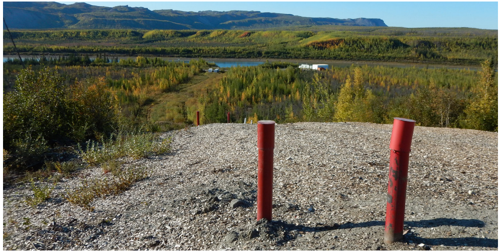
Slope monitoring instruments on the Enbridge Line 21 pipeline right-of-way near the town of Tulita, Northwest Territories. A variety of instruments are used measure ground movement in key locations along the pipeline.
