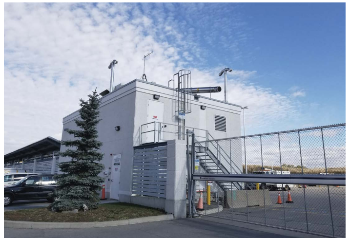
> Power-to-gas plant in Markham, Ontario
