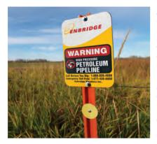
A pipeline follows a narrow, clear stretch of land, called a ROW, that allows our employees and contractors to access the pipeline for inspections, maintenance, testing, and emergencies. Approximate location of the pipeline can be determined by the pipeline marker. A few important notes when it comes to ROWs and pipeline markers:
