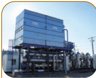
A new plant in Louisiana owned by Enbridge's Dufour Petroleum captures exhaust emissions from a nearby chemicals plant to produce food-grade CO 2 for use in carbonated products.
