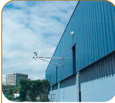
Enbridge Gas Distribution operates Solarwall technology at our Toronto garage facilities. By using solar energy to provide space heating, this technology has saved about 100 tonnes of CO 2 equivalent since its installation in 1999.
