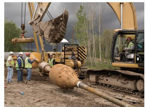
For large rivers or certain sensitive crossings, directional drilling is an appropriate and preferred construction method, depending on geologic conditions and other factors. HDD construction is considered suitable for large river crossings, extreme congestion (e.g. crossing rail yards), or other unique site-specific situations because it minimizes impacts on the area above the drill.
