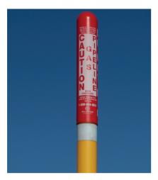
Pipeline markers do NOT indicate exact locations of a pipeline. Call or Click Before You Dig to have pipeline locations marked.
