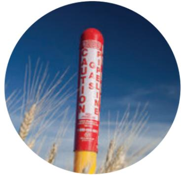
All pipeline markers provide important information including the pipeline owner name, the type of product being carried and an emergency number for reporting pipeline emergencies:
