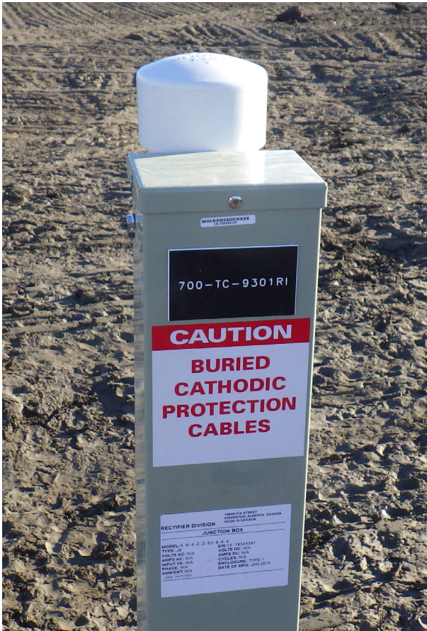
Enbridge personnel need infrequent but regular access to cathodic protection posts along our pipeline rights-of-way for inspection and maintenance.
