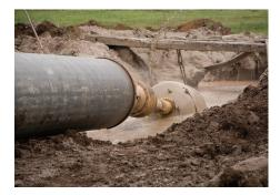
The length of time needed for drilling depends on the distance of the underground drill; the geology; the pipeline's diameter; and, the progress of drilling operations. Sometimes, drilling can be completed in just a few weeks. Other times it may take a few months to complete. Advanced planning can provide an estimated completion time for any specific drill site. These timetables, however, can be affected by unforeseen conditions.
