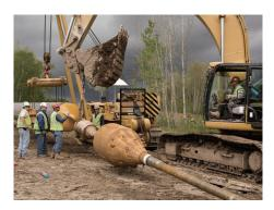
For large rivers or certain sensitive crossings, directional drilling is an appropriate and preferred construction method, depending on geologic conditions and other factors. HDD construction is considered suitable for large river crossings, extreme congestion (e.g. crossing rail yards), or other unique site-specific situations because it minimizes impacts on the area above the drill.
