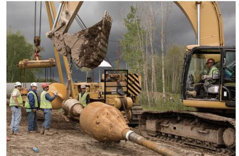
For large rivers or certain sensitive crossings, directional drilling is an appropriate and preferred construction method, depending on geologic conditions and other factors. HDD construction is considered suitable for large river crossings, extreme congestion (e.g. crossing rail yards), or other unique site-specific situations because it minimizes impacts on the area above the drill.
