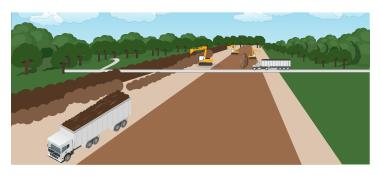
7. Trucks also haul in soil for backfill material to fill the trench.
