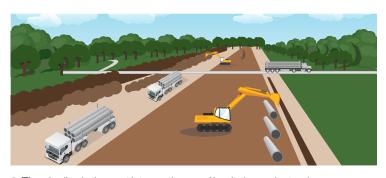
6. The pipeline is then cut into sections and hauled away by truck.
