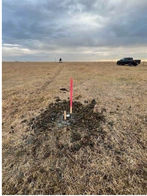
Photograph #69: Post-Drilling SS-BH25-56
