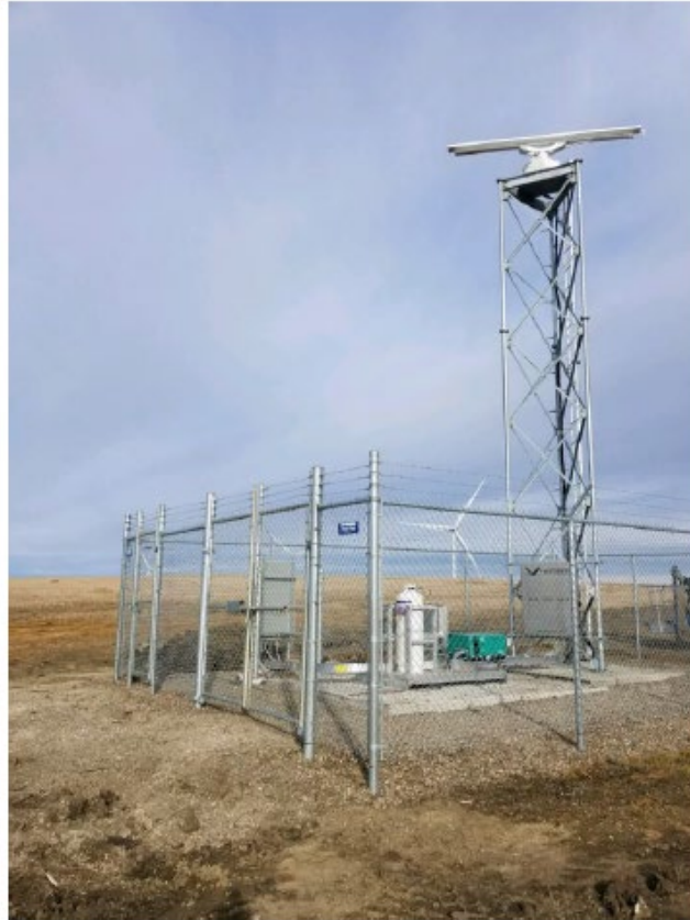
Figure 4: Image of a typical aircraft detection radar tower
