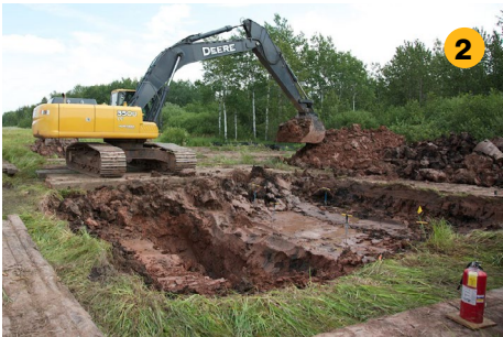
Excavate to expose the pipe
