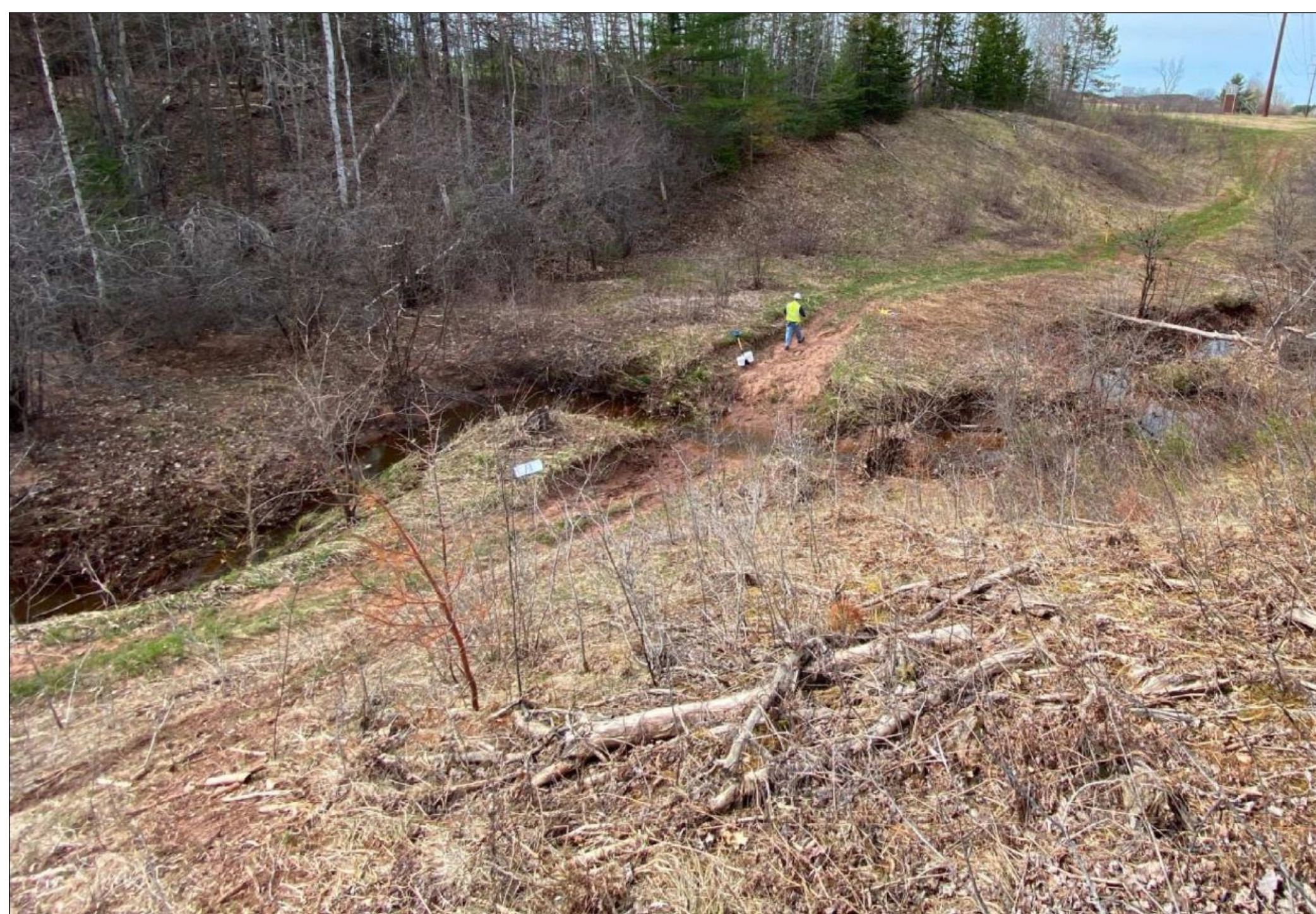
DOWNSTREAM RIGHT, EXISTING CHANNEL (NORTH BANK BACKGROUND, SOUTH BANK FOREGROUND)
