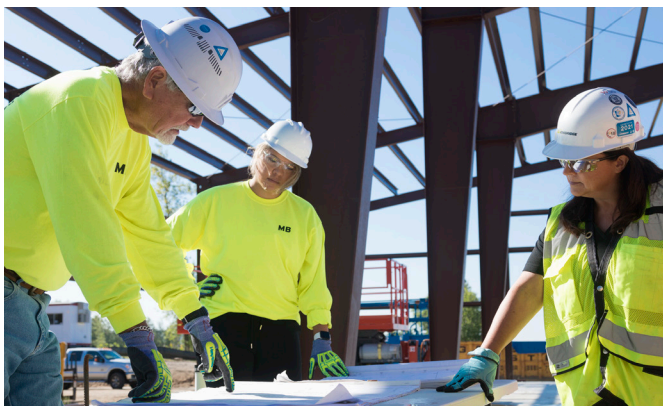
> Indigenous-owned MB Customs worked on the Line 3 Replacement Program in Minnesota.
