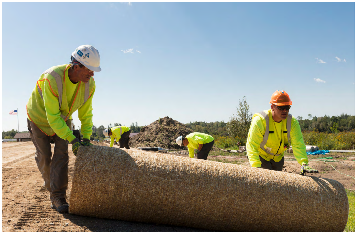
> Indigenous construction workers building the Line 3 replacement pipeline in the U.S.
