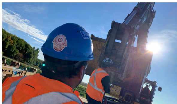
> Line 3 Decommissioning Canada.
