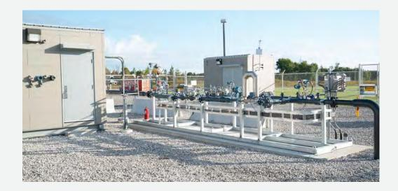
In January 2022, Enbridge Gas and our partner Cummins announced that North America's first hydrogen blending initiative was fully operational and serving the southern Ontario city of Markham. We now have the capacity to deliver blended gas – that is, green hydrogen injected into the natural gas distribution network to reduce the fuel's carbon footprint – to about 3,600 customers in Markham.
